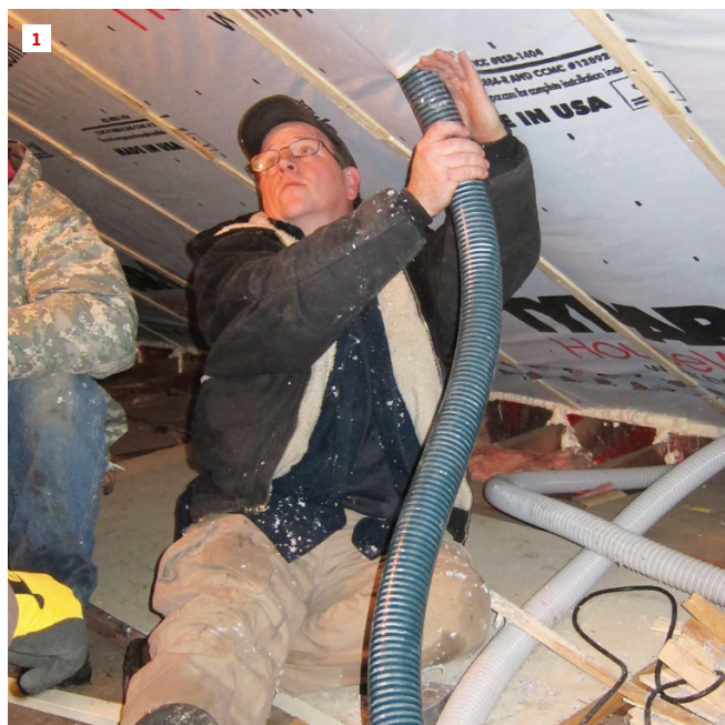
In existing construction, weatherizers typically dense-pack cellulose behind strapped housewrap (1).
