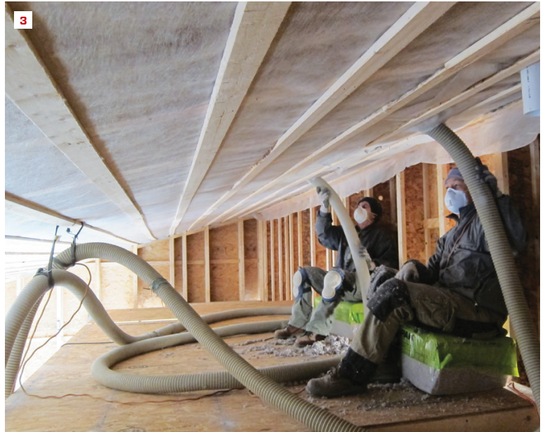
Where access from below is impractical, cellulose can be dense-packed into existing rafter bays from the roof ridge (2) . In new construction, the author recommends packing the material behind strapped Insulweb fabric (3) .
