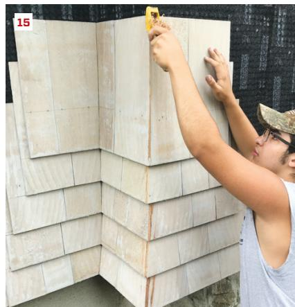
On the outside corner, the author uses a flexible batten to scribe the first starter shingle (11), then tacks the shingle in place and scribes the back of the opposing shingle (12). A Surform tool is used to smooth the joint after the second shingle is installed (13). Once the starter course is in place, the first course and subsequent courses are installed in similar fashion, working from the inside to outside corners (14, 15).
