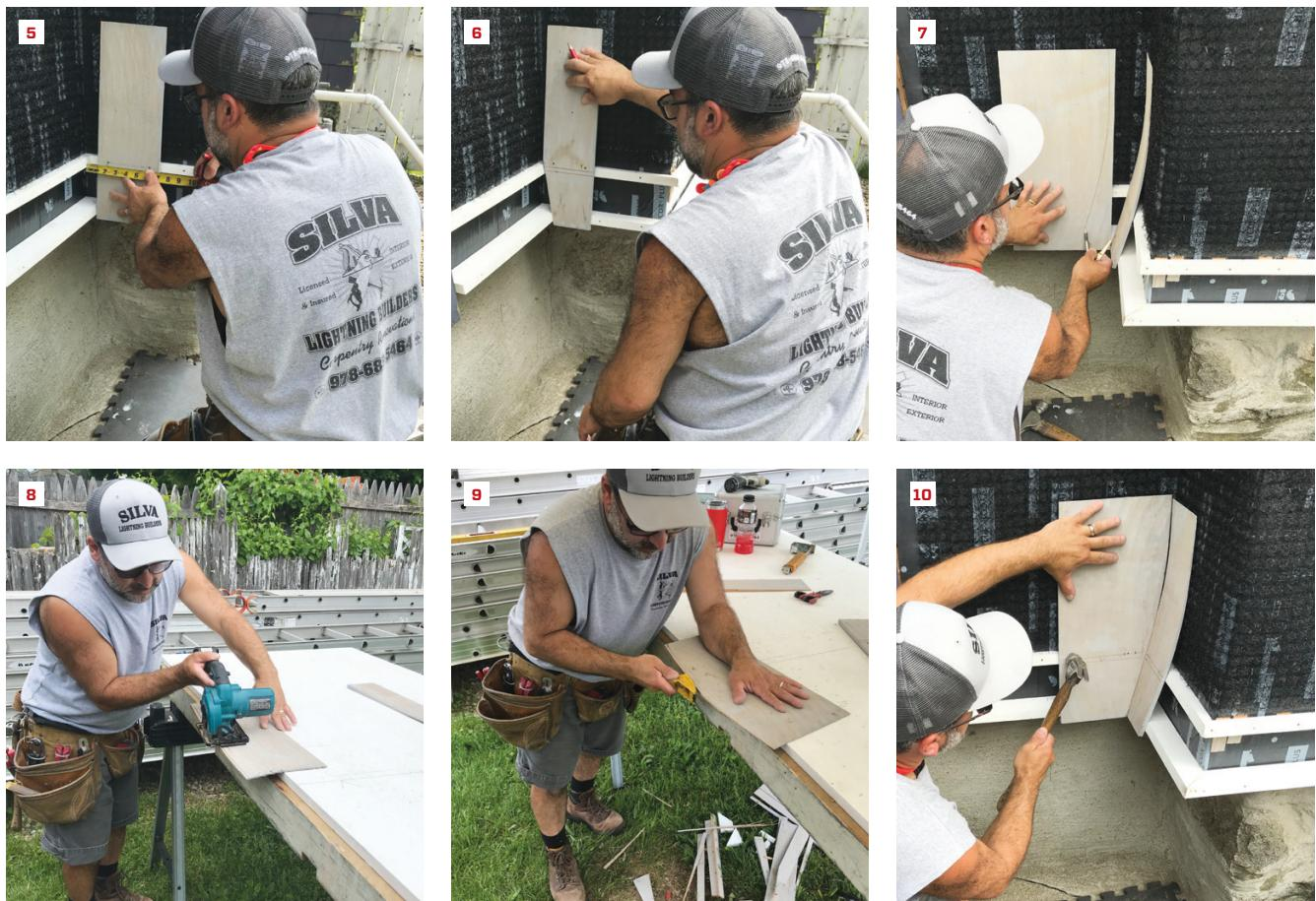
The author trims enough of the first inside corner shingle so that the edge is flush with the wall (5, 6), tacks the shingle in place, and uses a compass to scribe the flare on the opposing shingle (7). Then he cuts (8) and planes (9) the shingle to the scribe line before tacking it to the furring strips with 2-inch ring-shank siding nails (10).
