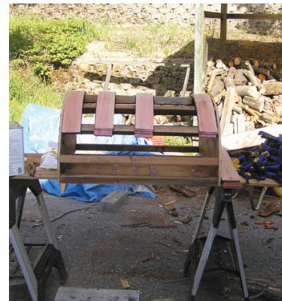
To laminate curved braces (similar to the arched subrails in the photo at top left), the author assembles plywood forms with 2-by stringers connecting the sides (above left). The stringers provide plenty of room for the multiple clamps needed to bend the laminations (above center). After the epoxy adhesive has cured, the clamps are removed (above right).
