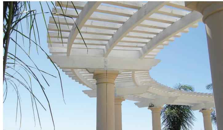
These arched subrails (above left) and sweeping pergola rafters (above right) are just two examples of how the author has incorporated curved laminations into his projects. Learning to glue together multiple thin layers of wood while bending the glued layers around a curved form is the key to making these elegant architectural details.
