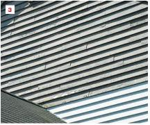
While the painters' work affects how good the paint job looks (1), what happens before they arrive affects how well the job performs over time. Bowed and buckled clapboards are often caused by interior moisture driving through siding that has not been back-primed (2, 3).
