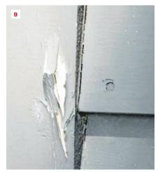
Here, carpenters have installed factory-primed window casing without sealing the ends. Failure has begun at unprimed ends (7), and in one case, water absorbed into an unprimed end has caused the wood to check (8). Not all of the failure is due to the carpenters, however. Stain was applied without any sanding or a second coat of primer, causing the finish to fail (9).
