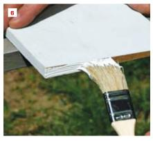
Unprimed siding won't hold paint for long. This paint job on a new addition (4) is less than five years old. Factory-installed primer is better than no primer, but it won't block the bleed-through of extractive oils in cedar (5). An additional coat of acrylic primer is needed before the finish coat. All field cuts need to be primed before installation of all siding and trim (6).
