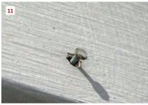
Water will collect and seep into the wood around an overdriven nail (10). Over time, smooth-shank nails will work their way proud of the surface (11) as siding changes in moisture content and temperature. Nails like this should be replaced with stainless steel, ring-shank nails.
