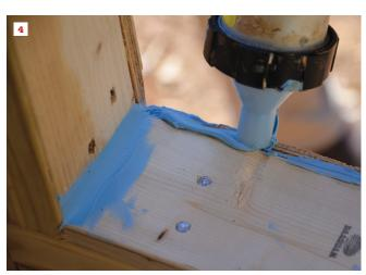
The roofing crew applies peel-and-stick underlayment to the plywood roof deck (1), rolling the material under pressure to create a good bond (2). The painters apply Joint Filler 2200 to sheathing cracks and nail holes (3), as well as to window rough-opening corners (4).
