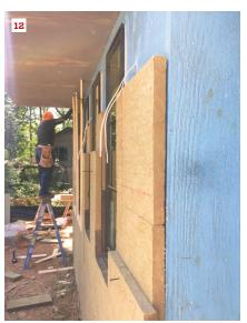
Outriggers are secured to the roof deck with structural clips (9), and the roof deck is insulated with Rockwool Toprock DD (10). The walls are insulated with Rockwool Comfortboard 110, with joints staggered (11, 12). The insulation is secured to the wall with battens and long screws.
