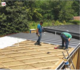
The shell has a continuous blanket of Rockwool (13). Strapping holds the insulation in place and provides nailing for the siding. The roofers install standing-seam metal roofing (14, 15). The siding crew installs Fry Reglet metal trim pieces (16).
