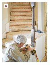
Workers removed the old rails and balusters, but left the turned newel posts in place (1), reinforcing them with pocket screws (2, 3). The landing newel post had to be relocated, so the author reinforced the connection with construction adhesive (4) and structural screws driven through the base of the newel post into the framing (5).
