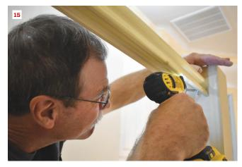
The author milled the poplar handrails in two pieces, then joined them using glue, Festool dominoes, and plenty of clamps (11, 12). A table saw fitted with a dado head was used to cut the baluster channel in the underside of the rails (13). For a precise fit between the stair newels, the author lay the stair rails across the treads to mark their length (14). After checking the fit, a worker drills holes for the pocket screws that will be used to fasten the rails to the posts (15).
