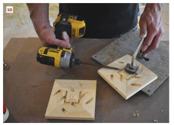
The crew used spacer blocks when clamping the sleeves to ensure they would fit over the old newels (6). A router with a flush trim bit was used to clean up the glue joints (7), while a 45-degree chamfer bit was used to profile the sleeve corners (8). The sleeves fit snugly over the old newel posts (9). Post caps were glued and pocket-screwed together (10).
