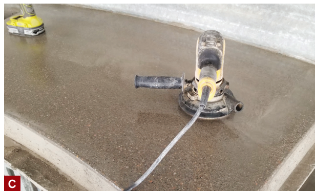
Figure 3. The author framed the kitchen cabinetry with light-gauge steel (A), then used cement board to form the base of the countertops, and smooth MDO plywood screwed to blocking to form the sides (B). Once the concrete cured and the forms were removed, the tops were polished smooth (C), then acid-stained and sealed with epoxy (D).
