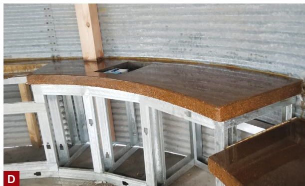
Figure 3. The author framed the kitchen cabinetry with light-gauge steel (A), then used cement board to form the base of the countertops, and smooth MDO plywood screwed to blocking to form the sides (B). Once the concrete cured and the forms were removed, the tops were polished smooth (C), then acid-stained and sealed with epoxy (D).
