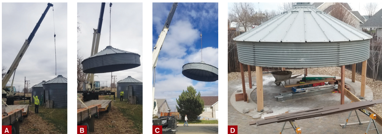
Figure 2. After most of the bolts holding the grain silo sections together were removed, a crane lifted the roof and upper section from the rest of the structure (A) and set it onto a flatbed trailer (B). At the client's home, the silo roof was hoisted over the house (C) and set gently onto temporary 4x4 posts. Later, permanent 6x6 posts were installed (D).
