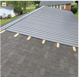
We place screw holes in the center of the pan, just to the right of the rib, and use 1-inch roofing screws to secure the panels (11). Ridge cap is secured to the ribs of roofing panels with stitch screws for a metal-to-metal connection. Typically, we complete the roof in sections (12) so we don't have to move ladders around the house multiple times and continually walk back and forth to one work station.
