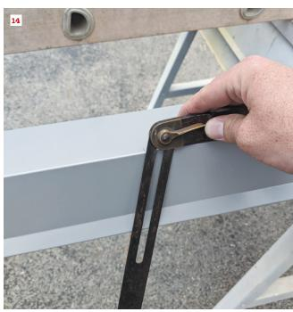
After the roofing panels are installed, we cover the gable edge with rake trim. To find the plumb cut for the trim at the peak, we use a sliding bevel square (13, 14); it's a simple, old-school tool, but it works well.
