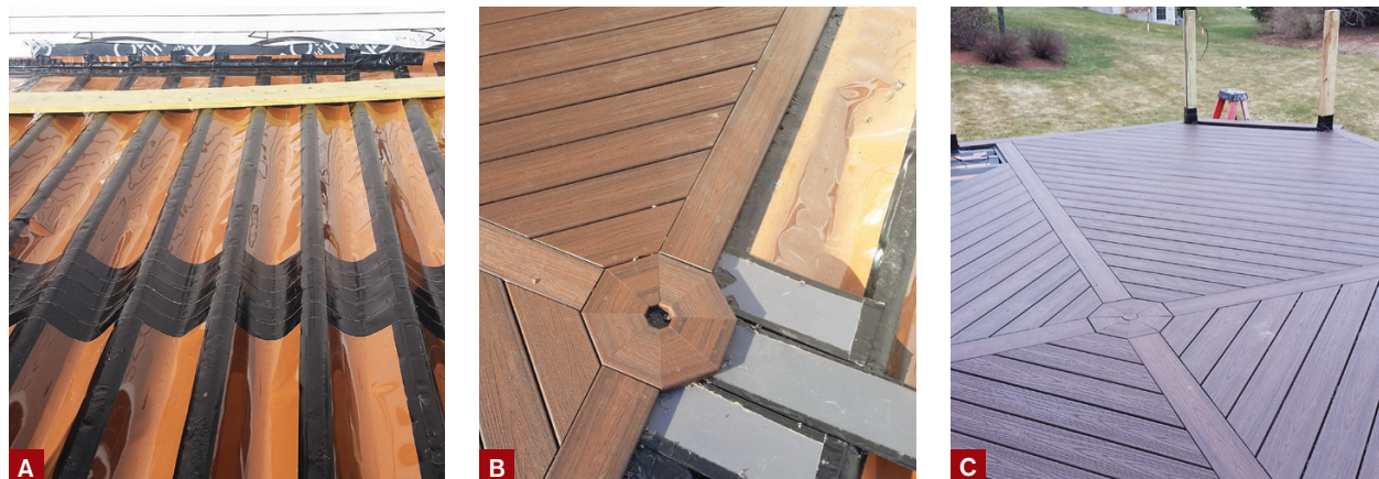
Figure 2. To keep the area below the deck dry, workers installed a Trex RainEscape under-deck drainage system (A). Extra courses of waterproofing tape underneath divider boards and over the blocking needed for the octagonal inlay protect the troughs from damage (B). After the drainage system passed water-testing, Trex decking was installed using hidden fasteners (C).
