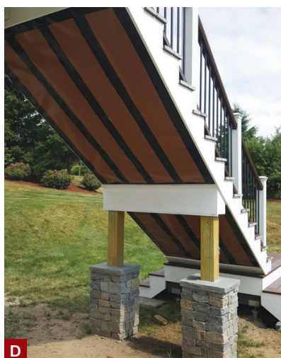
Figure 3. Workers determined the position and elevation of the stair landing with the help of a stringer for the upper flight of stairs (A). The landing was framed with steel and supported by helical piles (B). Steps lead up to the landing from all three sides (C). RainEscape troughs were fastened to the stair stringers so the underside of the stair could be finished with beadboard (D).
