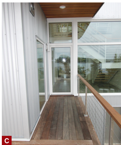
Figure 6. A custom-built guardrail with cable railing was installed (A). The deck was temporarily treated as two separate decks with code-approved guardrails (B, C). Guardrails and decking were reconfigured during the pavilion work (D).
