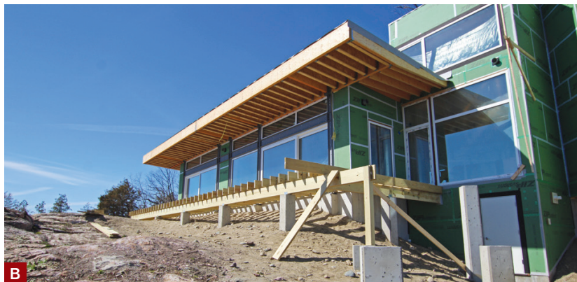
Figure 1. The bedroom-office wing was "floated" on the piers. Here, the deck was being framed on the home's elevated southeast corner (A). The larger deck off the main living area was close to grade and supported by shorter piers (B).
