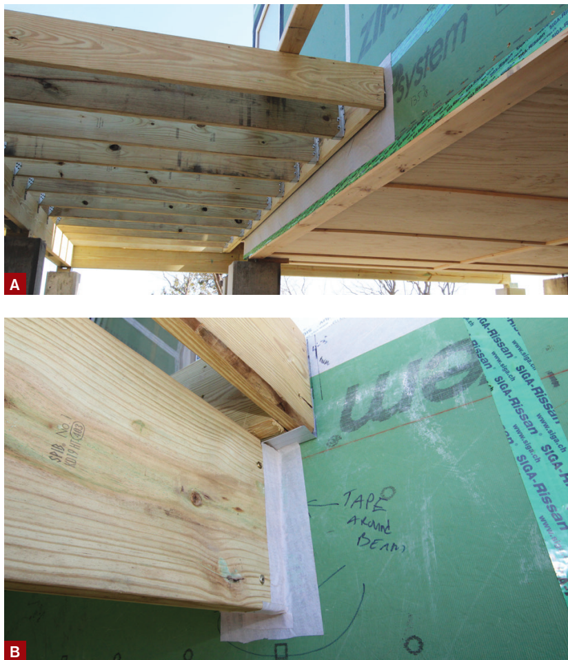
Figure 2. Ledgers were lag-bolted through spacers to the elevated floor's triple LVL rim beams spanning the piers (A). Fentrim flashing tape was used for both water- and air-sealing. Here, it air-seals a deck beam pocketed into a wall (B).
