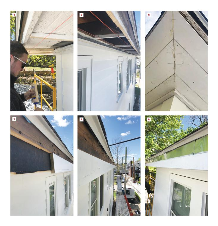
To accommodate the out-of-level eaves, new soffit was supported with tapered blocks in some areas (4), but in others, the old soffit was torn out and a new soffit plane was created with sistered framing (5). Three soffit boards allowed for some adjustment in width, but the boards had to align at corners (6). Part of the old fascia was left in place, ripped level, and joined to new fascia (7, 8). The joint between old and new is flashed with coil stock (9).
