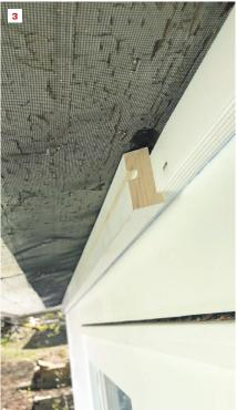
The author's sketch of the assembly he used to lay over the old eaves (top). He started with a line of 1-inch vent holes drilled through the existing soffit, over which he installed bug screen and Cor-A-Vent (2). He then milled a "frieze mold" from  $^{5}/_{4}$  stock with a rabbet to lap over the Cor-A-Vent and a groove to accept the soffit (3).
