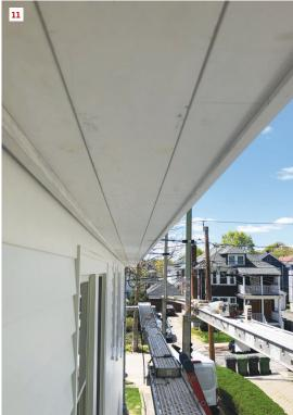
With nail holes filled and the new assembly painted out, the crisp lines of the new assembly come to light (10, 11). When completed with new gutter all around, the 100-plus-year-old home looks as straight and new as the day it was built. You would have no clue that old, multilayered, out-of-whack eaves were behind the new work (12).
