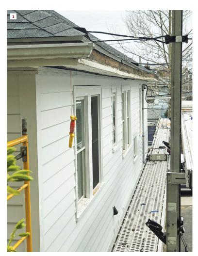
**Roller coaster eaves.** This house got an entirely new face lift, which included a tear-off and replacement of all the old siding and trim. But rather than demolish the eaves and rebuild them, the author chose to lay over the old eaves with a new assembly.
