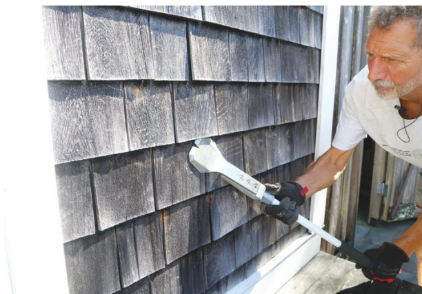
The salvage blade is useful for stripping siding (above left). Other blades include (above right, top row) finish nails; salvage; decking; 8-inch; and (bottom row) 3/4-inch; 1 3/4-inch; spike puller; 3-inch; 6-inch; and buried nail-head puller.
