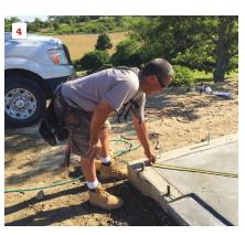
Start with a level foundation—no more than ½ inch out of level throughout the building. After confirming that the foundation walls are parallel (1), lay out and snap chalk lines for the mudsills (2). If the diagonal measurements for the opposing corners are equal, the foundation is square (3). If not, you'll need to adjust the wall layout until the diagonals are equal (4).
