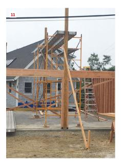
After the wall sheathing is nailed off, the wall can be lifted into place on top of the sill plate (here, the author is using wall jacks) (9); leaving the anchor bolts loose allows for adjustment as the remaining walls are raised. Diagonal bracing holds the walls in position (10) as the project moves into the next phase: roof framing (11).
