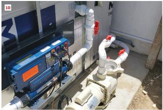
The hydraulic power unit is located away from the pool, set on a 2-foot-by-2-foot concrete pad, and shrouded in a rain cover. Access to both ends of the pool is required to maintain equipment (8). The galvanized steel panels are installed (9) with rigid insulation set in the bays. The unit is fitted with a "Gecko" water-quality/heat controller and filter motor (10).
