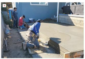
The preassembled unit's slab is formed up with the rebar installed (4). All the pool's mechanical equipment and metal frame panels need to be bonded together and grounded. Here, a Ufer ground is bonded to the slab's rebar (5). Concrete (3,000 psi) is pumped to the backyard slab (6) and finished off by the concrete sub's crew (7).
