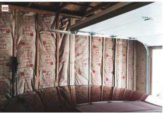
While fiberglass batts are noncombustible, their kraft paper facings are combustible. Whether located in a semi-enclosed space such as an attic (21), or in an open non-living space such as a garage (22), the paper facing should either be removed (or non-faced batts used) or be in close contact with drywall or another substantial material, rather than air, to reduce the risk of fire.
