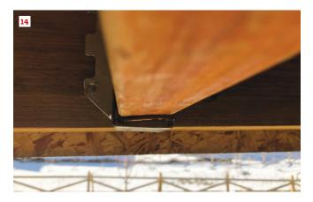
When the gap between a supporting framing member and a truss or sawn joist supported by a joist hanger exceeds <sup>1</sup>/s inch, either between the two framing members **(12, 13)**, or between the framing member and the joist-hanger saddle **(14)**, the hanger's published load capacity no longer applies and must be reduced according to tables published by the hanger manufacturer.
