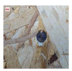
There should be a ½-e-inch gap between sheathing joints, which should occur over the centerline of the framing, with nails installed per the recommended nailing schedule and ½ inch from the panel edges (seismic and wind zones require closer spacing) (18). Depending on how many overdriven nails there are and how deeply they are embedded in the sheathing, they may reduce the shear capacity of a panel (19, 20).
