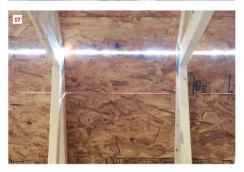
Sheathing that doesn't span more than two rafters or joists (15) as required by code can't adequately support a concentrated load. When sheathing is between 16 and 24 inches wide (16), the edges must be supported by clips or blocking; solid blocking is required with narrower panels (17).
