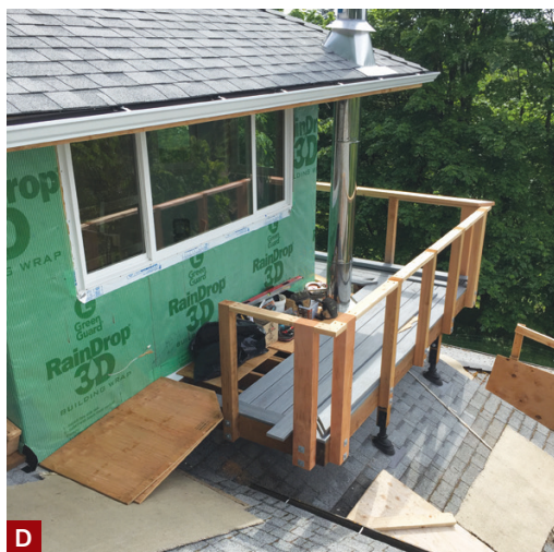
Figure 3. Part of the wrap-around deck is supported by cantilevered beams (A), with the rest bearing on beams supported by 4x4 PT Doug fir posts bolted to SkyLift risers (B). After bolting 4x4 and 4x6 clear cedar guard posts to the framing (C), the crew installed a 2x4 subrail and began installation of the capped composite decking that would complete the project (D).
