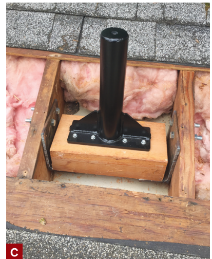
Figure 2. The crew opened up the roof sheathing and bolted steel angle brackets to the roof framing (A), with 4x6 Doug fir blocks bolted to the steel angles (B). SkyLift risers were then bolted to the blocks to help support the deck (C).
