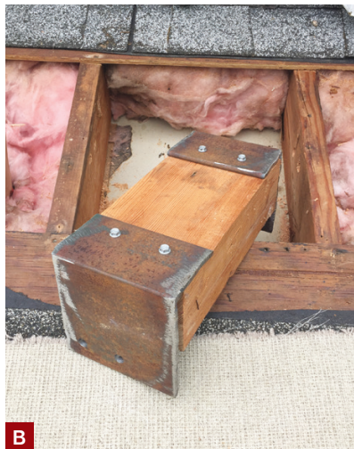
Figure 2. The crew opened up the roof sheathing and bolted steel angle brackets to the roof framing (A), with 4x6 Doug fir blocks bolted to the steel angles (B). SkyLift risers were then bolted to the blocks to help support the deck (C).
