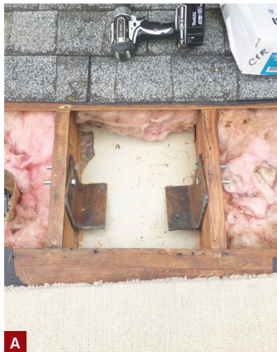
Figure 2. The crew opened up the roof sheathing and bolted steel angle brackets to the roof framing (A), with 4x6 Doug fir blocks bolted to the steel angles (B). SkyLift risers were then bolted to the blocks to help support the deck (C).
