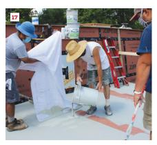
To dry-in the large solar roof project, workers applied base coat and fabric to the Zip System sheathing seams (12). Zip tape was used to seal a roof-to-wall intersection (13). After spreading out the tack coat with a roller (14), workers bedded fabric in the coating (15), then applied the saturation coat (16), taking care to smooth out wrinkles in the fabric (17) as they squeegeed the coating to the desired 25-mil thickness.
