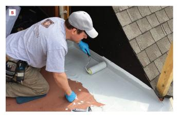
Instead of sealing the sheathing joints on this small upper-story deck with Zip tape, which would telegraph through the Acrylabs coating, workers troweled on a smooth layer of Sikaflex sealant (1). Before applying the Acrylabs tack coat, the reinforcing fabric was carefully cut to fit (2), then rolled up for later application. The coating can be applied by brush (3, 4) or "squeegee-style" with a  $^{1}$ /2-inch nap slit foam roller (5).
