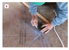
A full-scale drawing allowed the crew to visualize the intersection of the radial rafters. After swinging a semicircle to represent the top plate (3), they used a ripping to trace the rafters one by one (4). Darkening the lines let them see the end cut details (5).
