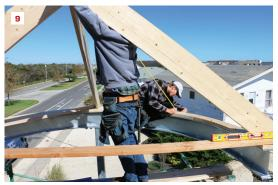
The crew found the midpoint of a 2-by spanning between the common rafters and transferred that point to the plate to mark the positions of the "eighth" rafters (6). Midway between those points and the common rafters (7), they marked the positions of the "sixteenth" rafters (8). After laying out the rafters, the crew measured from the plate to the shoulder of the angled cut to find the length of each rafter (9).
