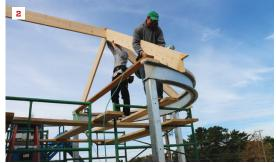
Like framing a hip roof, framing a cone begins with three common rafters. The first comes off the end of the ridge (1), and the other two support the ridge from the sides (2).
