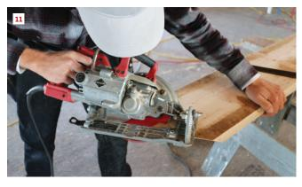
The rafter tails were identical to the commons, so the crew used the pattern rafter to trace the tail, and then cut the details (10). After measuring and marking the shoulders of the plumb cut, they took the saw angle from the floor drawing and cut the top (11).
