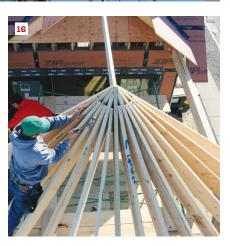
The arcs between the king commons were each a fourth of a circle's circumference. The first two rafters installed split those arcs into eighths (12). Starting at one end of the semicircle, the crew then installed the four rafters that created sixteenths along with the eight "thirty-second" rafters (13, 14). They nailed the rafters together at the peak (15) and tapped down any uneven ones (16).
