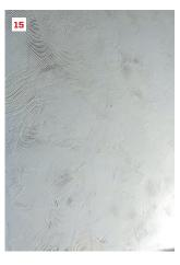
On this small crack, helper Derek Dawson uses a putty knife to flatten the new plaster and push it in along the edges (11). The electrical box is set at the proper depth to avoid interfering with the new finish (12). The lime-putty coat is applied in two passes; here, the first pass is made (13). Ron Bisson uses a texture comb to mimic an existing swirl pattern (14, 15).
