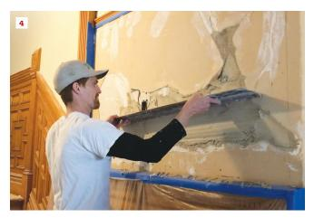
Built in 1884, the mansion had a number of different plaster finishes. Here, Ron Bisson applies brown coat to a textured wall using a putty knife (1) and a trowel (2). Pushing the brown coat hard against the old plaster helps key it in along the edge (3). On large repairs, a 42-inch-long slicker is used to flatten the brown coat using a sawing motion (4).
