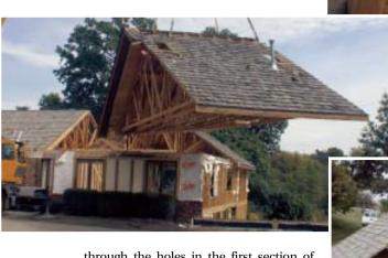
through the holes in the first section of roof, wrapped them around the LVLs, and used shackles to connect them to the lifting straps. After the crane operator lifted
