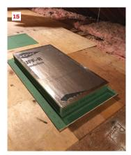
The author shimmed the apron level (11) before screwing it to the attic floor, then sealed the gap between the floor and the apron with foam (12). Before installing the hinges, he screwed a pair of blocks to the apron (13) to allow the hatch cover to remain open without a separate prop (14) and to close snugly without pinching the gasket on the hinge side of the cover (15).
