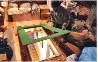
After fitting the foam top and sides (5) to the hatch cover, the author taped all the joints with foil-faced HVAC tape (6) and applied a gasket to the bottom edge of the cover (7). Next, he assembled (8) and installed (9) the foam jamb extension that lines the stair opening. Before installing the apron, he applied a zigzag bead of foam insulation to the floor of the attic around the opening (10).
