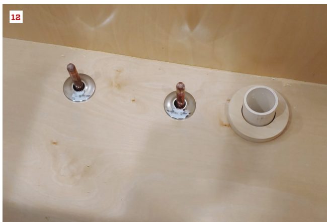
A jig speeds installation of cabinet hardware (10). When a cabinet that has already been drilled for plumbing lines has to be shifted slightly, a wood trim ring can be fabricated to cover the enlarged hole around a drain line (11, 12).
