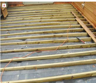
When installing decks over living space, the author adheres to a code-mandated minimum 1/4-inch-per-foot roof slope, which can be achieved by either sloping the roof framing or using a tapered insulation system. While uniformly deep 2-by "floating" sleepers laid across a sloped roof may be installed (1), most clients prefer a level walking surface, so sleepers are typically tapered (2).
