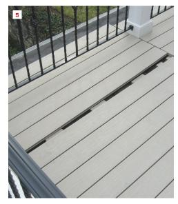
Though not usual, sleepers may be fastened to 2-bys laid on the flat, which helps distribute loads over a wider area (3), particularly when a protection board is not installed between the roof membrane and insulation or when a roof insulation with a lower compressive strength is used. Removable access panels are recommended on the deck above both the high and low ends of the roof (4, 5), to provide access to the roofing membrane for maintenance.
