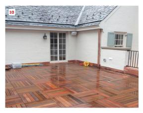
Pedestal supports are well-suited for roof systems with multiple slopes, including tapered roof-deck insulation sloping towards scuppers for drainage (6). Most pedestals are adjustable and are supplied by their manufacturers in varying heights depending on the roof configuration (7). Installation is a simple matter of following the manufacturer's layout and adjusting the pedestals so that they are level with each other (8) as each paver (9) or decking panel (10) is installed.
