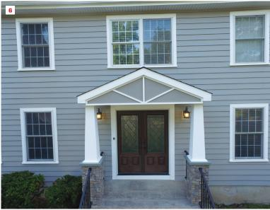
For a brief time, Marvin **(5)** made siding from pultruded fiberglass—the same material as in its Integrity windows. Azek **(6)** made a similar type of siding. Both companies offered 7-inch-exposure clapboards, for which there is high demand. This was a superior siding material most notably because boards could be butted to trim and no caulk was necessary when they were properly flashed. The look was perfection. Unfortunately, both products have been discontinued.
