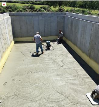
While this slab on an older project uses wire mesh, the author has gravitated towards using fiber-mesh reinforcement to simplify the pour. Both will provide good reinforcement but must be coupled with saw-cut control joints (after finishing) to avoid cracking. With a solid base, reinforcement, and proper curing, the author avoids any visible cracks in the slab surface.
