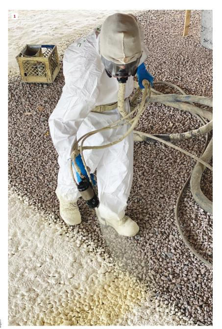
Two inches of closed-cell spray foam provides not only good insulation but also a superior air and water barrier. The author has found that spray foam works best when applied over a compacted crushed-stone base.
