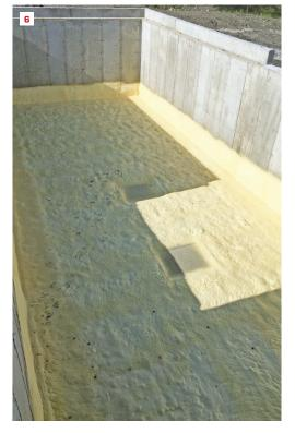
Elevation lines on this foundation wall show the layers of the typical basement slab for the large custom homes built by the author (2). Over the compacted gravel subbase, crushed stone is spread and compacted smooth **(3, 4)** before the foam is applied (5). Note the foam is brought up the wall **(6)** a good 12 to 16 inches to get it well above the slab surface to tie in with the wall insulation and ensure a continuous seal.
