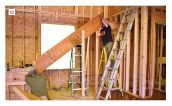
OSB sheathing was glued and screwed to the inner faces of the short walls (5) supporting the landing platform, which was framed with 2x12s (6, 7). Workers then installed blocking and a temporary support ledger (8) for the upper landing (9), which was propped up and held level with temporary posts (10) while the LVL stair stringers were measured, cut, and installed (11).
