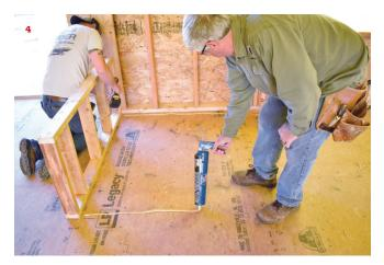
To preserve the home's symmetrical fenestration, the stairs needed to be spaced away from the wall (1). The author began by marking the stair's vertical layout on a story pole, including each tread (2) and the landing elevations (3). Plenty of structural screws and construction adhesive were used to frame each landing (4).
