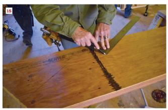
The author used the story pole to mark the tread locations on the inside stringer (12). Because the inside and outside stringers were solid instead of notched, 2-by blocking was glued and screwed to the stringer to support the treads (13). Then the author transferred the tread layout to the outside stringer using a spirit level and a straight 2-by (14). The middle stringer was also cut from a 16-inch-wide LVL, which needed to be notched for the treads and risers (15).
