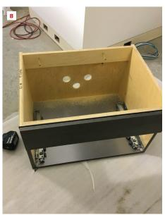
Working from the inside, the hole saw punches through the finish face (7). Here, the holes for the supply lines were cut larger to accommodate shut-off valves installed on the stub-outs; valves are typically installed after the cabinet installation (8).
