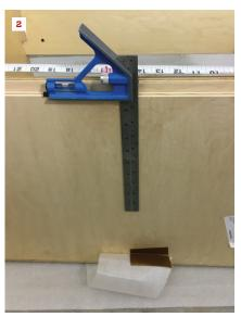
After accurately aligning cabinet cut-outs with roughed-in plumbing, the author assembles a "floating" vanity, (1). A "reference" centerline is marked on the cabinet's back panel with a combo square (2).
