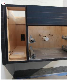
The example vanity cabinet installed. A 1/2-inch hole was made to run power to an outlet on the side of the vanity (9). More typical, "tighter" 3/4-inch holes were cut for 1/2-inch supply-line pipes in another vanity unit (10). Also, an electrical box was cut inside the cabinet (electrical boxes are similarly measured, though cutouts are made with a multi-tool or jigsaw).
