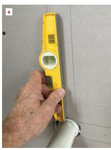
After marking outside lines with a torpedo level, the author measures between the two lines to find dead-center. Here, he uses same increment either side of the 4- and 6-inch marks to find centerline, represented by the 5-inch mark (3). The torpedo level is used to make a centerline (4).
