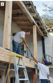
The new balcony-level 6x6 posts were slotted and bored to receive concealed post tie connectors (7). After the new 24-foot-long glulam was set in the beam saddles (8) and the posts installed, they were chamfered to match the original beams.
