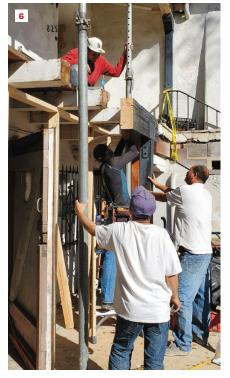
To provide level bearing for a temporary shoring to support the clay tile roof, sloped blocking was nailed into place (4). To remove the existing posts, workers cut the toenailed connection between the beam and the decorative capitals (5). The existing glulam was cut into sections prior to removal (6).
