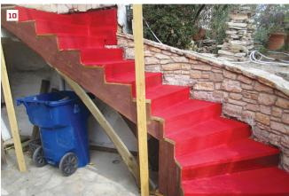
The new stairs were built with pressure-treated 2-by stock and PT plywood with compatible screws (9). Then the framing was sealed with a liquid-applied waterproofing and crack-prevention membrane (10).
