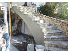
To prevent water intrusion, flashing that runs up the framing was sealed to the masonry (11). Then the stairs were papered and lathed with stucco wire on the stringers (12) and with rib lath underneath (13) prior to the application of a traditional two-coat stucco finish (14).
