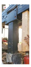
Installed in the 1970s, the existing glulam had rotated outward due to rot (1), causing a "hinge joint" to open up between the top of the posts and the decorative wood capitals (2). A 30-ton jack was used to separate the beam from its saddle-bracket connector (3).
