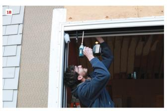
The doors will ride on the top track, so it's critical the track is level and securely fastened to the header. For this, the crew sets up a rotary laser (16), then drills the header for the lag bolts (17) and drives the bolts home with an impact driver (18). Note that the holes in the top track are angled towards the framing; this slight angle must be maintained when pilot holes are drilled.
