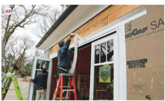
Each door panel is tilted to set the bottom guide into the track (19). The carrier hinge at the top is secured to the door with the supplied screws (20), and the bottom hinge secured to the door and guide at the bottom (21). A door jack helps set the door at the right elevation. When all the panels are installed, the author checks the alignment (22) and adjusts as needed, before the last steps: flashing the side jambs and, finally, the head flange (23).
