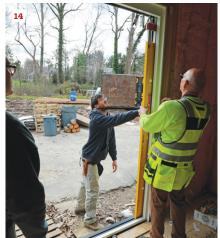
With the frame assembled, it is dry fit (11) and checked to make sure it will sit plumb in the opening (12). The crew then tips out the frame so the flange can be caulked (13). Even though the flange will be flashed with peel-andstick, caulk is still required by the door maker. Once sealed, the frame is again checked for plumb in all directions (14) and the diagonals checked that they're equal (15, facing page), before the flange is screwed off.
