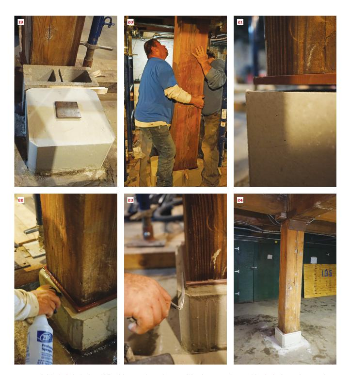
A 4x4 steel shim (19) sits in the middle of the new pier as the crew slides the cut post into position (20). The gap between the top of the pier and the setting plate (21) is soaked with water (22) before being filled with non-shrinking grout (23). Then all that's left to do is to remove the shoring around the completed post (24).
