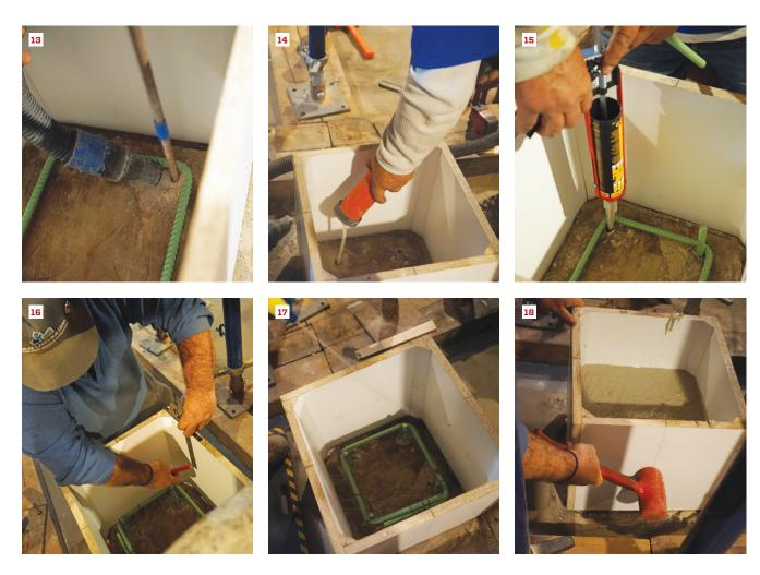
The crew drills into the existing footing for rebar pins (13). A vacuum, a wire brush, and a blow-out pump (14) are used to clean the holes before the pins are set with epoxy (15). The pier elevation is marked on the form with a combination square (16) and the form sprayed with water (17). Tapping the form with a dead-blow mallet settles the concrete and helps eliminate voids (18).
