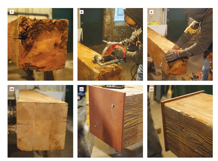
With the old post on sawhorses (7), the author uses a beam saw to cut off the rotten end, cutting to full depth on all sides (8) and finishing the cut with a handsaw (9). On the fresh end (10), he attaches a 12-by-12-by-1/2-inch steel setting plate (11, 12).
