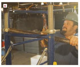
The existing footing was sound; only rot at the base of a post was of structural concern (1). A single layer of 4x6 cribbing (2) supports the shoring. Two towers—each made with two frames and topped with two steel beams—flank the post to pick up the load on the main girder (3, 4), while two ladder frames, one each on opposite sides of the post, pick up the loads on the intersecting joists (5). With the shoring complete, the crew tightens up the U-heads (6) to remove the load from the post.
