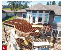
To complete the curved detail on the top deck (A), a custom-fabricated steel girder (B) was required. Bolted to the deck framing and house (B, C), the girder doesn't require a support post (D).
