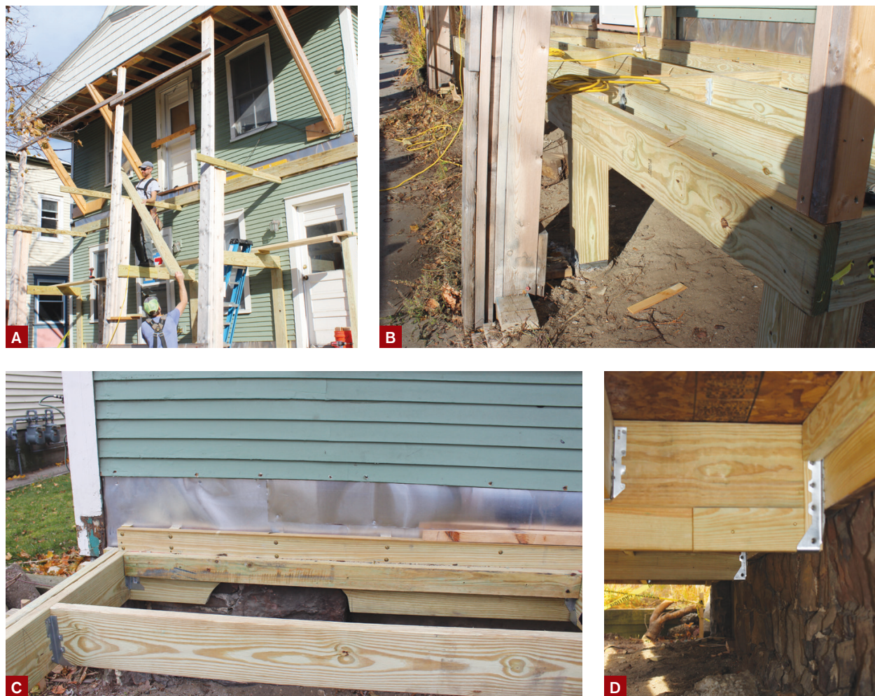
Figure 1. The author shored up the porch roof, then hired a demo company to remove the existing two-story porch (A). The new porch was conventionally framed with pressure-treated lumber, with the joists parallel to the front of the house (B). The oversized ledger was blocked out away from the wall (C) to clear the house's irregular stone foundation (D).
