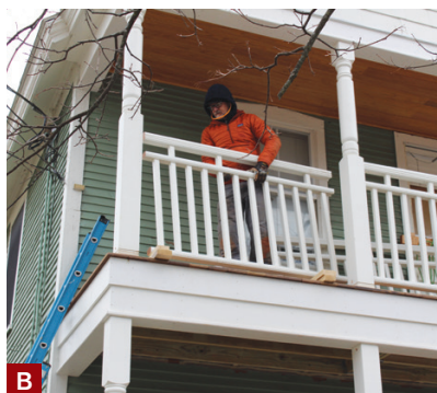
Figure 6. After cutting the rail sections on site to fit, Sean Laughlin sealed the end grain with primer (A) and then fastened the rails to the posts with structural screws (B). Making the railing connection at the house was complicated by the existing siding and trim (C).
