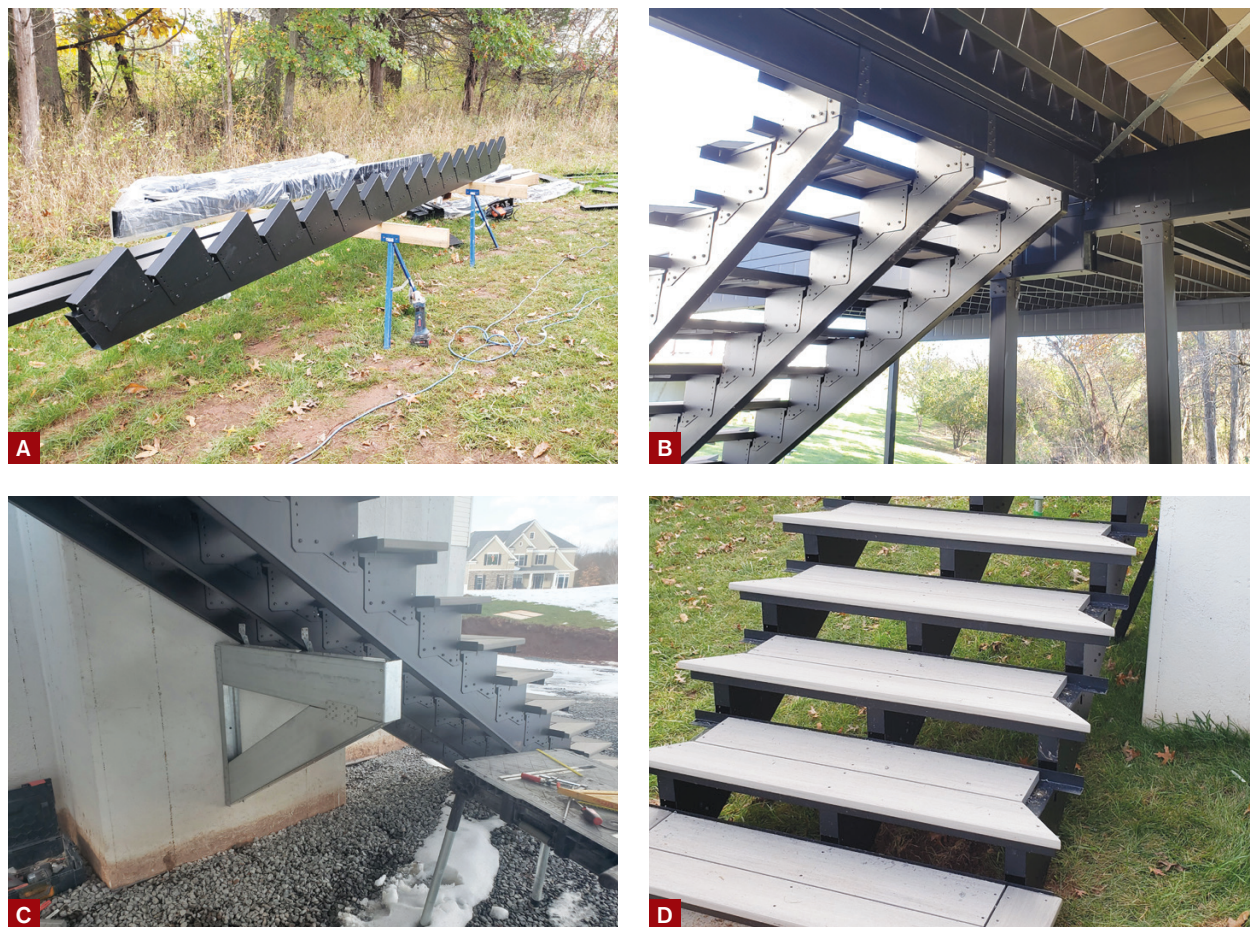
Figure 6. To build stair stringers, proprietary brackets are fastened to standard joists (A), which are then fastened to the framing with adjustable strap-like hanger brackets (B). A midspan bracket enabled the author to build the stairs before the hardscaping was completed (C). Wider, 7-inch deck boards created an overhang for the two-board treads (D).
