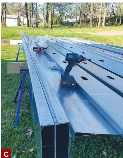
Figure 2. Evolution support posts are sized to fit standard 4x4 PT post hardware, such as the U-shaped helical pier brackets used on this project (A). The beams measure 2 inches by 11 inches and can be fastened together with tracks at both top and bottom to form double beams (B). The author found that the tracks—which can also be used with the joist material, but are available only in 4-foot lengths—made multi-ply beam assembly more labor-intensive than with LGS framing (C) and added to the size of double beams and joists.
