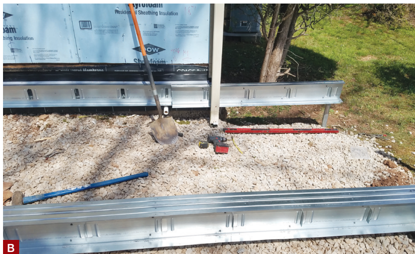
Figure 1. In the Evolution system, ledger brackets are screwed to the S-ledger, or fit into punched openings in the S-ledger without requiring additional fasteners (A). In comparison, an LGS ledger track has bent tabs for fastening the joists to the ledger (B) and requires five or more fasteners per joist-to-ledger connection. Evolution joists just slip over the brackets, and are held in place with a pair of screws per bracket (C).
