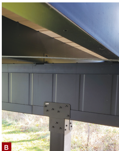
Figure 2. Evolution support posts are sized to fit standard 4x4 PT post hardware, such as the U-shaped helical pier brackets used on this project (A). The beams measure 2 inches by 11 inches and can be fastened together with tracks at both top and bottom to form double beams (B). The author found that the tracks—which can also be used with the joist material, but are available only in 4-foot lengths—made multi-ply beam assembly more labor-intensive than with LGS framing (C) and added to the size of double beams and joists.
