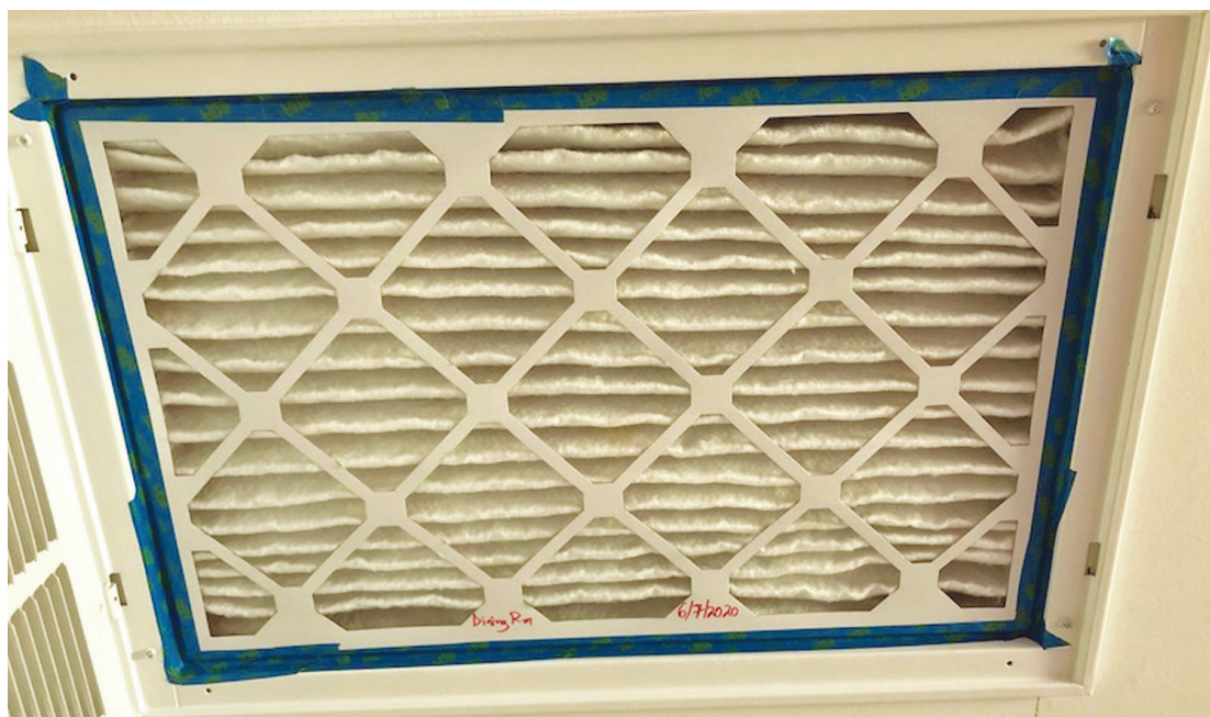
This 16x25 MERV-13 filter in a ceiling filter grille keeps the resistance low and the indoor air quality high.
