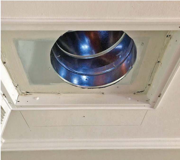
A shallow return (above) filter grille box results in a higher pressure drop across the filter. Replacing it with a deeper box (right) behind the filter succeeded in reducing the filter pressure drop by 30%.
