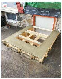
The author and his son, Carter, mixed up more than 50 bags of concrete on site (10), using shovels and a long pole to push the concrete to the bottom of the forms and eliminate voids (11, 12). Raised several inches above the level of the driveway, the new curb will block rain and snow from entering the bulkhead entry (13).
