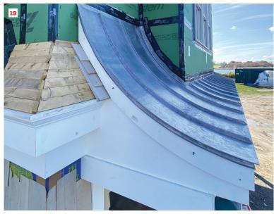
The standing seam is completed with a roofer's anvil and mallet, with the long leg on the second panel folded over the bent rib on the first (15). Once the seams are folded together, they are pressed tight with tongs (16). At the transition between the metal roofing and the wall, the top of the pans are folded over (17) to prepare for seaming them to a horizontal strip of transition metal (18). The top edge of this transition flashing is taped to the sheathing with Zip System tape (18, 19).
