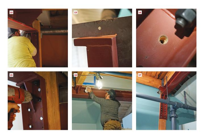
With the beam secured, a crew member lifted one end bracket into position (12). Note how the bracket was purposefully fabricated out-of-square to accommodate the out-of-plumb column (13). Each bracket required 20 lag screws, and each hole for the lag screws was predrilled using two different drill bits—one sized for the threaded shank and one for the shoulder of the lag (14). The crew alternated holes when driving the lags (15). As a final step, the beam was wiped clean (16, 17).
