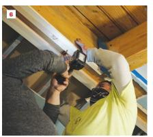
The author's crew set up scaffolding and craned the replacement beam onto the top lift (1), positioning it in front of a window (2). Note the gusseted flanges on the left side of the beam; these were added to support the purlins (3). Once the demo crew had cleared the site, the author set up shop and began ripping leveling strips (4), which his crew screwed to the bottom of the failed beam (5, 6). These strips would provide a level surface against which they could place the new steel beam.
