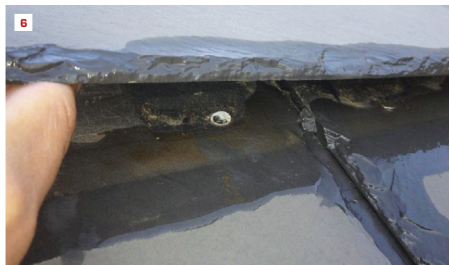
Installing slate without the correct overlap can allow water to wick under the shingles and corrode fasteners, particularly on low-pitched roofs (6). Also, long-lasting fasteners should be used; electro-galvanized nails corrode quickly if they stay wet.
