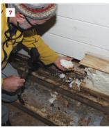
Seams in the sheet-metal bed had not been air-sealed, providing cold, moist air access into the framed floor (5, inset). More critically, warm, moist air from the interior condensed on the metal bed, saturating vapor-open batts; water accumulated in the batts over time, resulting in rotted OSB subfloor and framing (6). The problem was more acute along raised, uninsulated edges (7).
