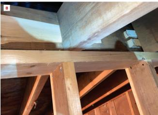
The framed wall that supports the rafters (7) is put together with screws—installing those proved much easier than trying to swing a hammer or use nail guns in the tight attic space. For good measure, the author shimmed any remaining gaps between the rafters and the ridge board (8).
