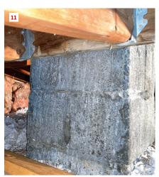
Rafters abutting a header at the block chimney had dropped (9). We jacked those individually (10) and attached the rafters to the header with joist hangers (11).
