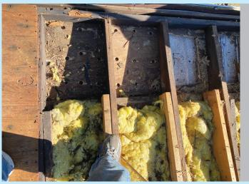
Where sheathing was completely loose and needed to be replaced, we took the opportunity to add cellulose insulation (photo, top left). Note: This end of the house has a cathedral ceiling with insulation between the rafters. It was designed, in fact, with a ridge beam. The exterior walls in this area did not spread.
