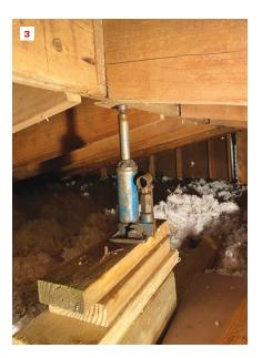
One sign that something was wrong was a slight dip in part of the ridge that was visible from the exterior when the roofing was stripped. Inside the attic, the problem was much more apparent: One ridge board had dropped approximately  $1^{3}/4$  inches (1). Along the ridge board, some of the rafters had pulled away (2). Remediation began with jacking the ridge board back in place (3).
