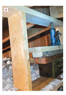
Initially, the author cut temporary support blocks from 2x4s and posted them down to a center bearing wall (in line with the center girder supporting the first floor) (4). The final solution was to build a short wall, starting with top and bottom plates (5), then jacking the top plate up as much as possible to push up any rafters that had dropped down (6), before infilling with short studs.
