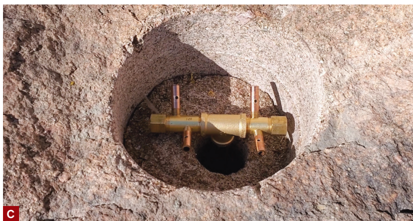
Figure 3. Along with the burners installed in the two boulders, there are also two ground-level burners (A). The black steel gas supply lines run through 2-inch-diameter holes drilled through the boulders (B). Rated at 50,000 Btu each, the assembled brass burners will be covered by porous lava rock (C).
