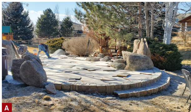
Figure 4. The fire feature is the cornerstone of a larger patio project (A), with multicolored flagstones set in mortar on top of a steel-reinforced concrete slab (B).
