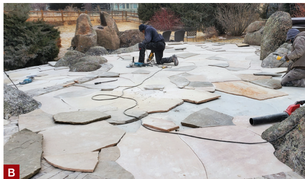
Figure 4. The fire feature is the cornerstone of a larger patio project (A), with multicolored flagstones set in mortar on top of a steel-reinforced concrete slab (B).
