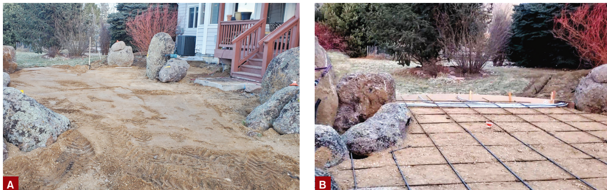
Figure 1. After laying a gas line in a 30-inch-deep trench and placing boulders in their proper locations (A), workers prepped the area for the concrete slab that would provide a base for the flagstone patio (B).
