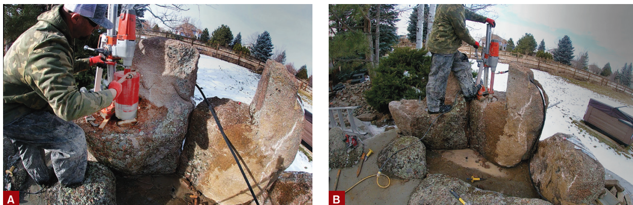
Figure 2. The author carved 8-inch-deep recesses into the tops of the boulders with a 10-inch-diameter core bit to house the burner assemblies (A). Then he drilled 2-inch-diameter holes down through the recess to connect to holes drilled horizontally through the backs of the boulders for the gas lines (B).
