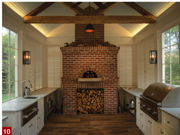
Beadboard is installed between trusses made from salvaged hand-hewn timber (9). The wood-fired oven is the focal point of the interior, which also features Carrera marble countertops installed on base cabinets and custom-fabricated stainless steel shelving (10).
