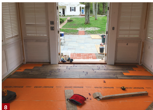
The custom-built windows and louvers are fitted with casement-window-style operable brass hardware. Here, hinge locations are routed out using a Porter-Cable hinge template (7). Porcelain tile that looks like hardwood flooring is dry fit over a Ditra uncoupling membrane (8).
