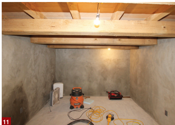
The wine-room walls are finished with a three-coat stucco finish (11). Designed by the architect-client, the wine shelving was built by NDC crew members using walnut-veneer plywood with walnut face frames (12).
