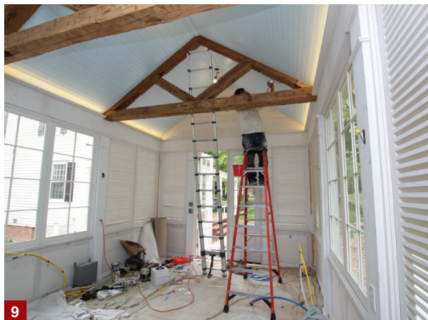
Beadboard is installed between trusses made from salvaged hand-hewn timber (9). The wood-fired oven is the focal point of the interior, which also features Carrera marble countertops installed on base cabinets and custom-fabricated stainless steel shelving (10).
