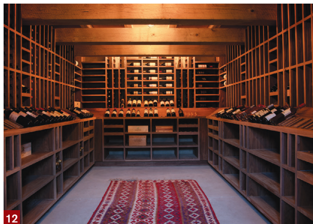
The wine-room walls are finished with a three-coat stucco finish (11). Designed by the architect-client, the wine shelving was built by NDC crew members using walnut-veneer plywood with walnut face frames (12).
