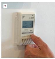
Ten wall-mounted units (4), six ceiling cassette units (5), and one concealed-duct unit supply conditioned air to the offices. An "intelligent Touch Manager" (6) controls the overall VRF multi-split system, while thermostats (7) in each office allow for localized control.
