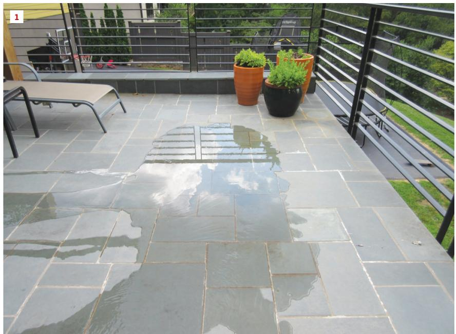
As shown on this exterior deck over habitable space, inadequate drainage caused by the deflection of a low-slope roof can lead to ponding.
