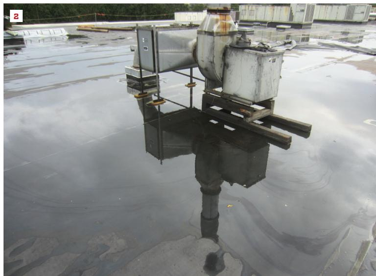
Roof deflection caused by the weight of mechanical equipment that wasn't accounted for in the original design can lead to ponding.
