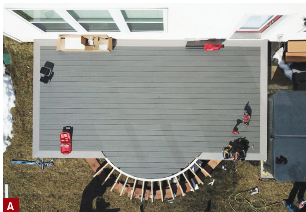
When installing the decking, the author avoided using any hidden fasteners where the inlay would be located (A). After tracing the inlay's outline, he cut out the decking with a small circular saw and pressed the inlay into place (B).
