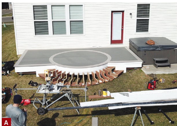
The stair stringers were fastened to the curved PVC rim joist with HeadLok flat-head structural screws, driven from behind through the rim into the stringer stock (A). The extra-wide treads consist of a double row of 1x8 decking (B).
