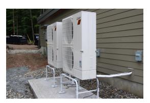
Heat pump stands, commonly installed today for cold-climate heat pumps, also reduce the likelihood of rodent damage; mice have difficulty climbing the thin factoryfinished legs.
