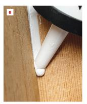
Two ways to cut the tip: a square cut (4) and opposing angle cuts (5). Note that on the angled cuts, one cut is deeper than the other; they are not symmetrical. The author prefers to push the gun (6), keeping a small, raised puddle of caulk in front of the tip while he lays down an even, well-bedded bead.
