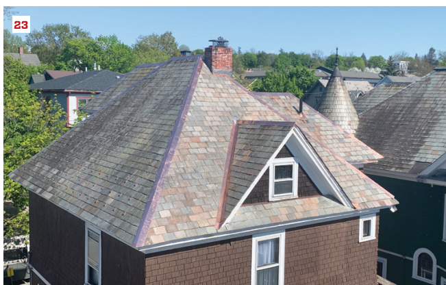
Salvaged semi-weathering green-gray slate blends into the existing slate on a finished open valley (21), dormer (22), and north- and west-facing sections of roof (23). Seventy-five percent of the existing slates were left intact.
