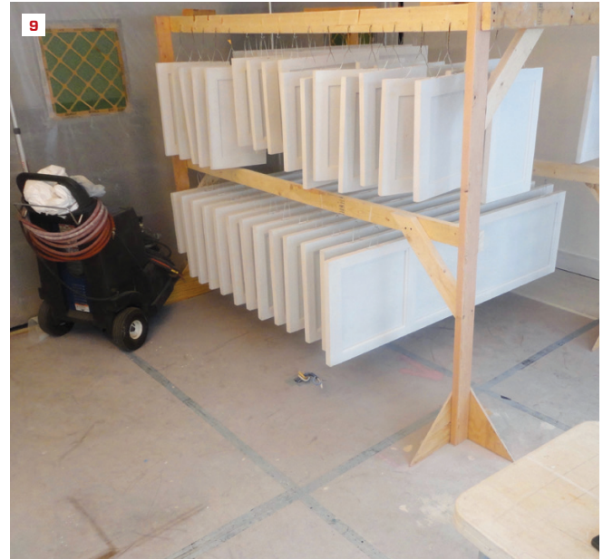
After the author sanded, stained, and finished the floor in this master bedroom (8), the room was used as a spray booth for cabinet doors during the course of the renovation (9). Fully taped hardboard over paper protected the flooring.
