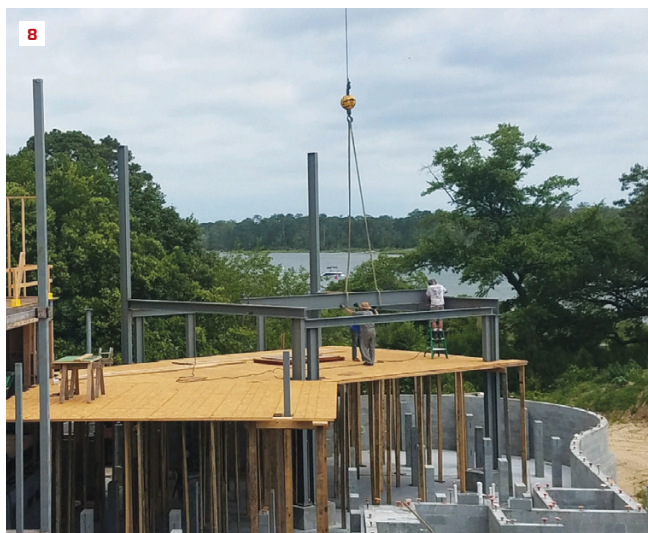
The framing crew erected an extensive temporary scaffolding system over a future outdoor living pavilion to install the complex steel framing for the master suite (8).
